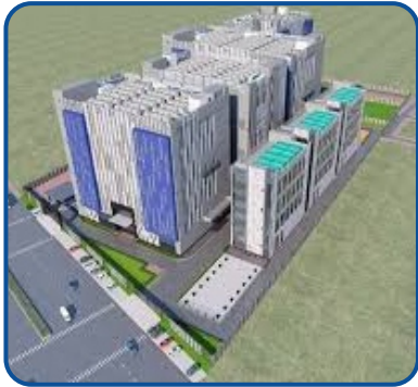
Piling for BAM DLR Data Centre, URC Construction
